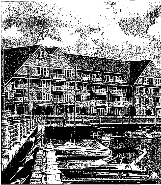
Cape Cod shingle-style architecture graces the 40-unit Atwater at Gaslight Pointe, a condominium community within walking distance of downtown Racine.
